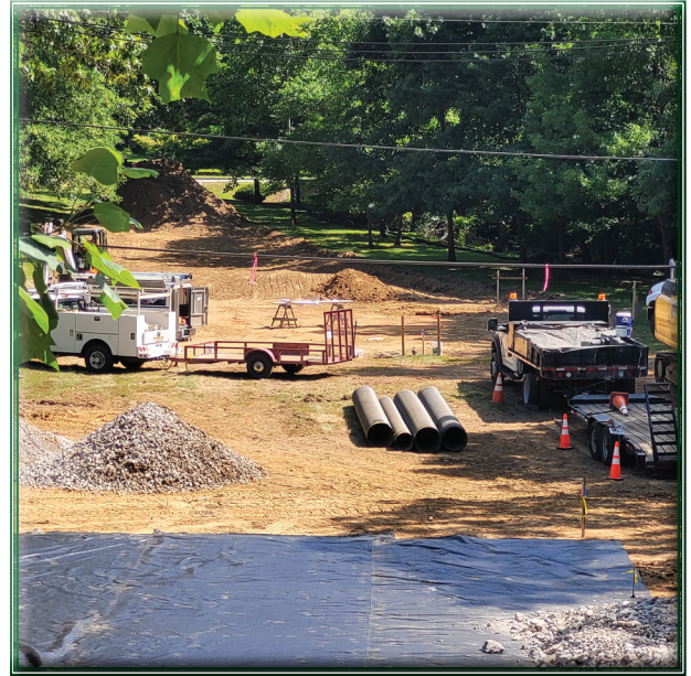
Construction has started on the Little Hunting Creek Improvements.
